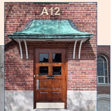
Refinished rectory door
