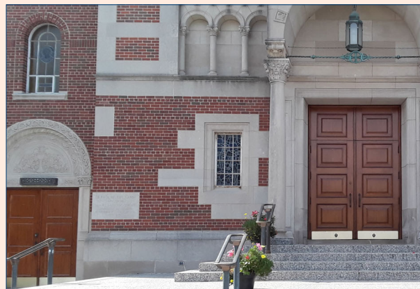
Refinished doors of Upper Church (view from Northwest Highway)
